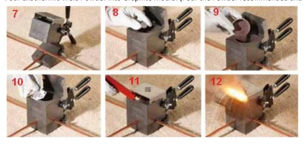
STEP - 10: Empty 50% of the starting powder above Exothermic Weld Powder (**Don't Mix, just scatter**) and then Close the Mould Mouth and then the rest 50% Starting Powder, sprinkle it on the Mould Mouth nearby the small hole given on the top of the Mould Mouth.
